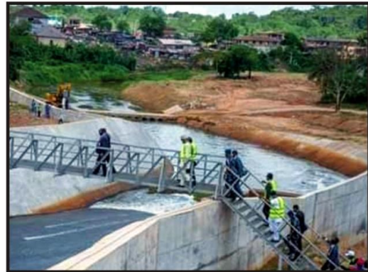
Improved Eleyele Water Dam
